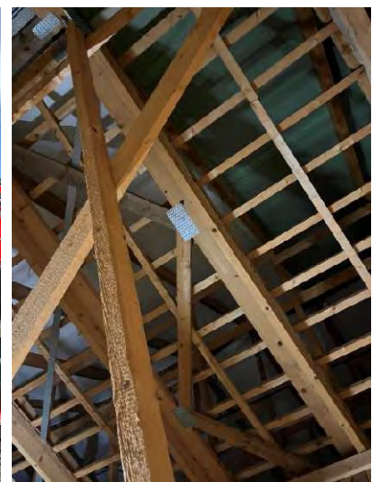
Nagelplattenbinder in Discounter
